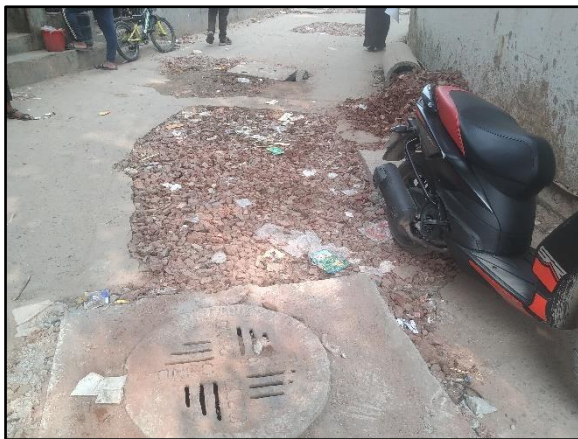
Figure 3: Broken carriageway
